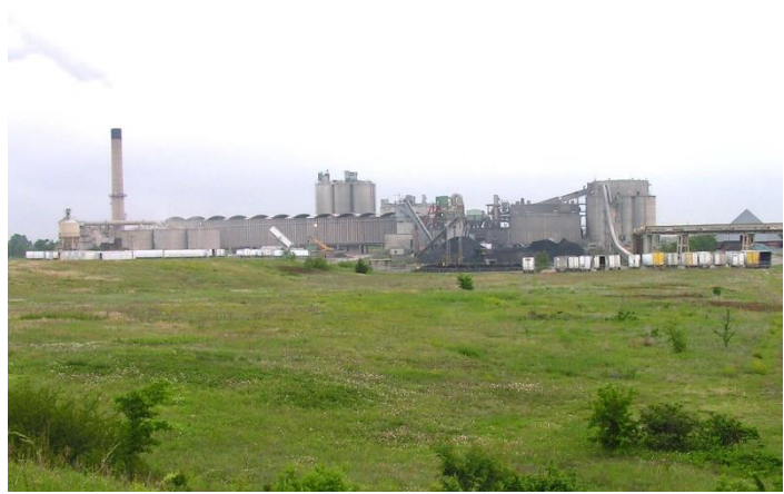
Holcim Inc. Cement Plant
